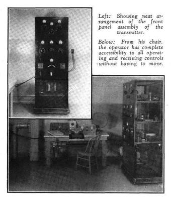
The receiving and transmitting apparatus is so situated that the operator may control the entire equipment from his seat at the operating table.
